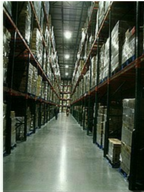
AFTER Energy-efficient LED requiring fewer fixtures & providing higher quality light.
